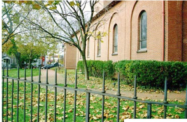
EXISTING BUILDING — VIEW FROM SIDEWALK, SOUTH
